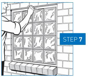
The last block does without one side having a PVC infill, insert a thin tip of the silicone gun and put a blob of silicone into the centre of the void. In the top joint, slide the PVC infill from the top of the neighbouring blocks so they are shared [using a screwdriver for example]. Check the alignment of the blocks and tap flush if necessary then allow a few hours for the silicone to cure.
